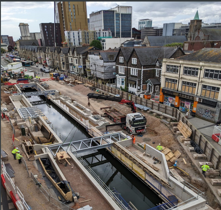
footbridge steelwork in place
