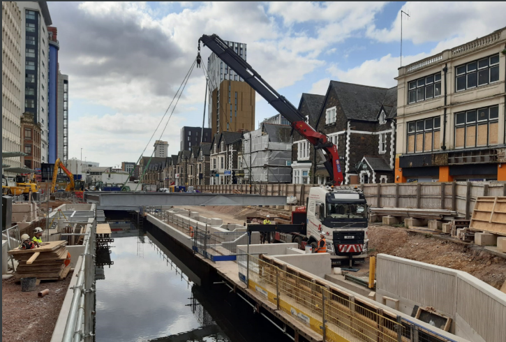
Installing steelwork for the footbridges
