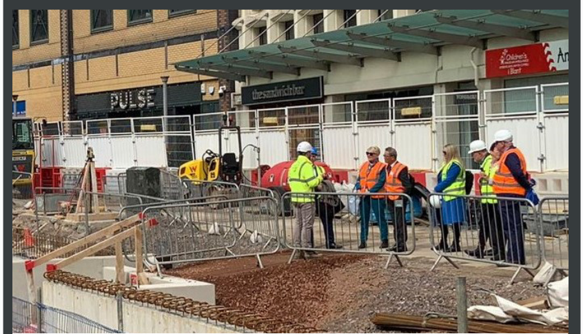
Site visit at the Canal Quarter
