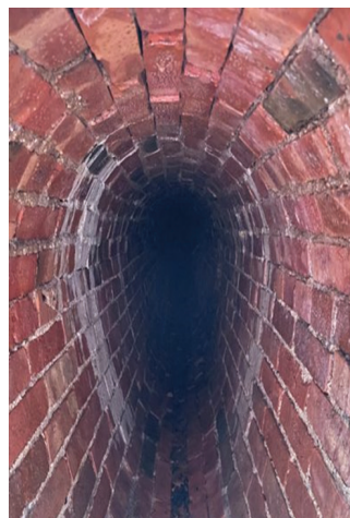
Old Victorian brick egg sewer on Queen Street
