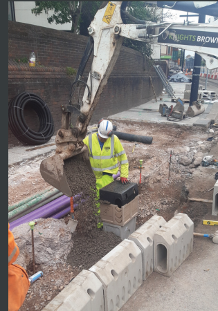
Installation of gully on Station Terrace
