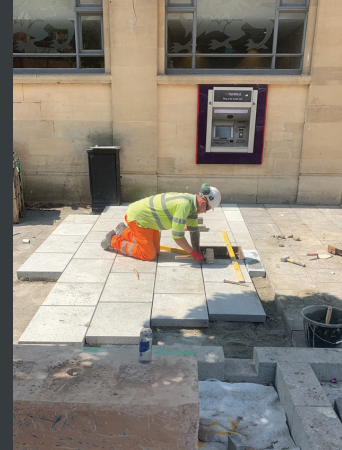
Laying new paving on Churchill Way
