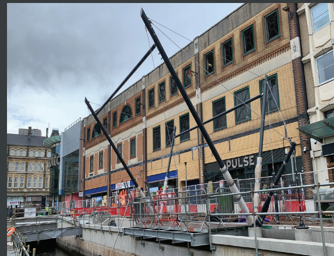
Base Structures Canopy frame installation
