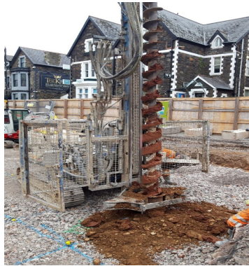
Piling works for the cantilever walkway
