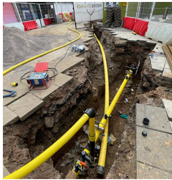
Utility diversions being completed at Canal Quarter
