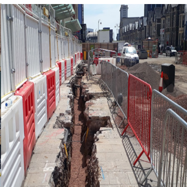
Gas & water main diversions
